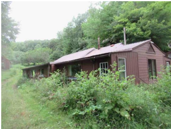
Main House – to be razed
